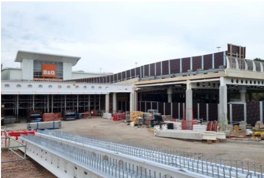
Castlepoint Car Park 2022 Kier Construction Health and Safety Ambassador Award
