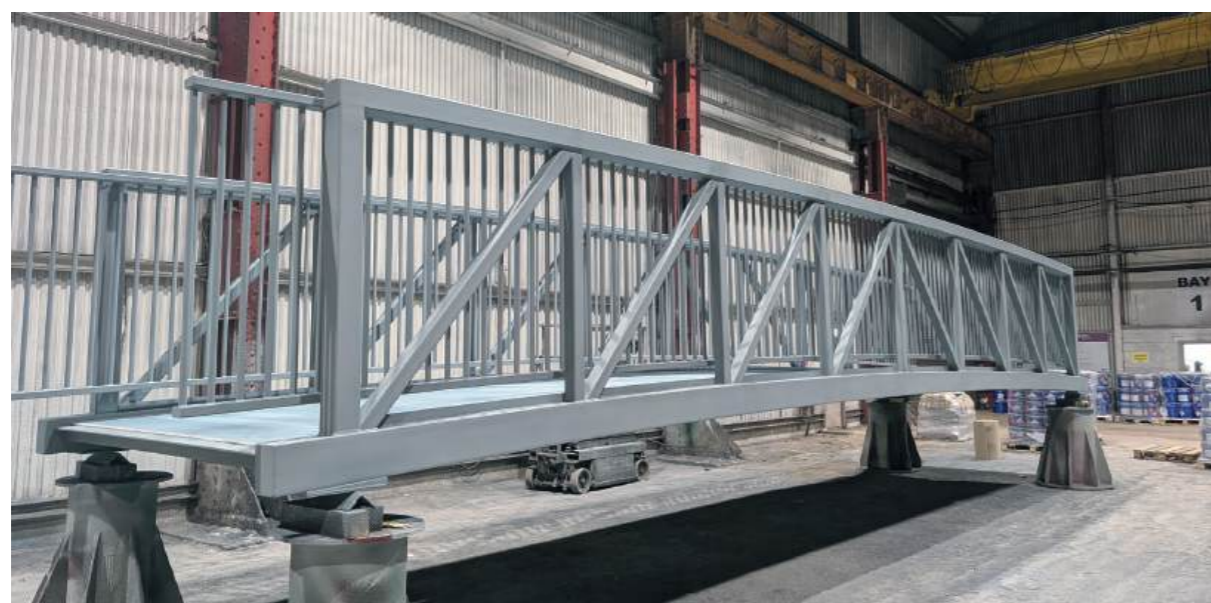
Cuckoos Hollow Footbridge, Peterborough
