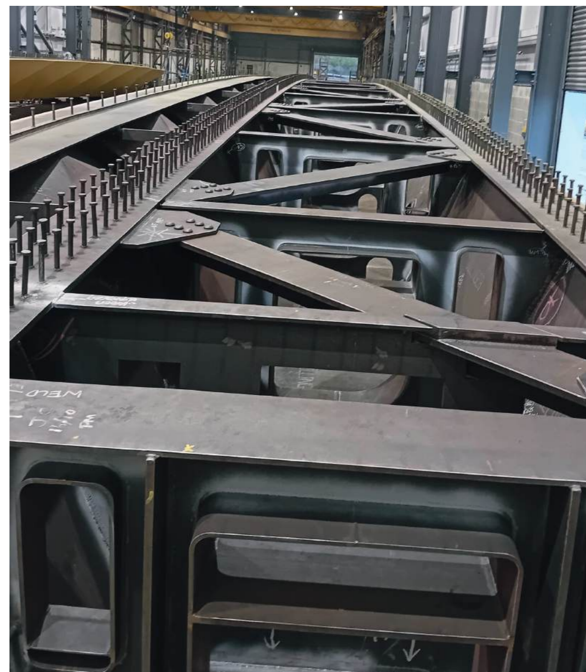
Meridian Water Bridge, in fabrication
