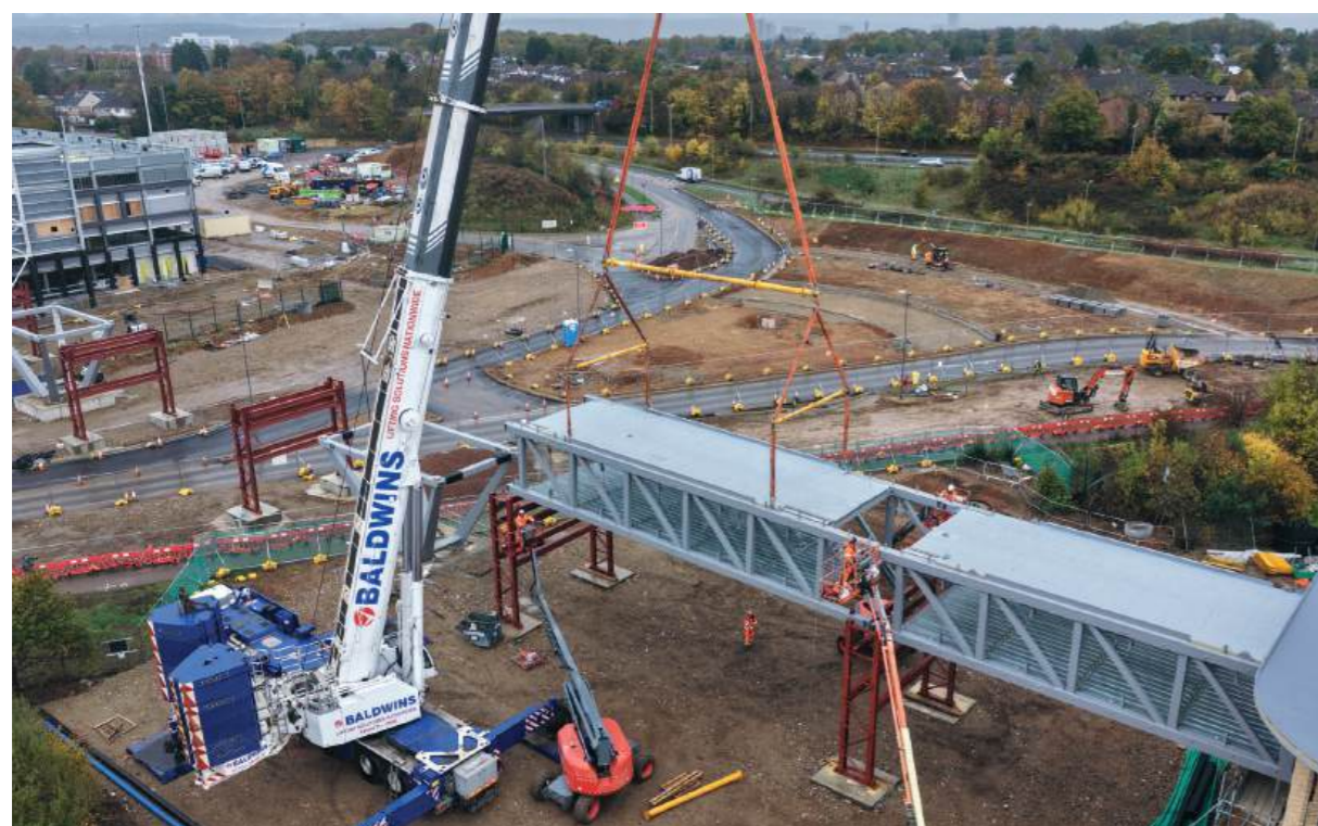
Project Merlin Footbridge Installation, Watford
