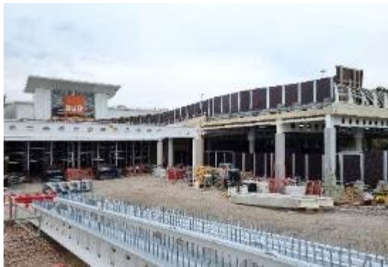
Castlepoint Car Park 2022 Kier Construction Health and Safety Ambassador Award
