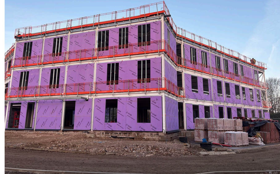
Medical Centre, Square One Construction
